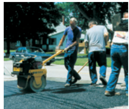
Single drum design delivers optimum maneuverability for patch work.
