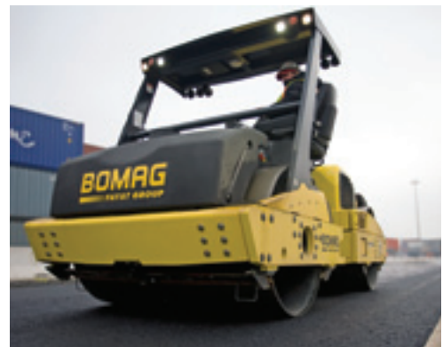
BW278AD-4 in action on asphalt
