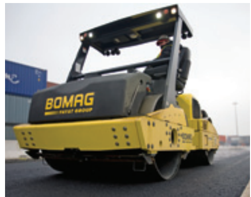
BW278AD-4 in action on asphalt
