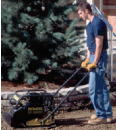
BP25/48D at work on soil application
